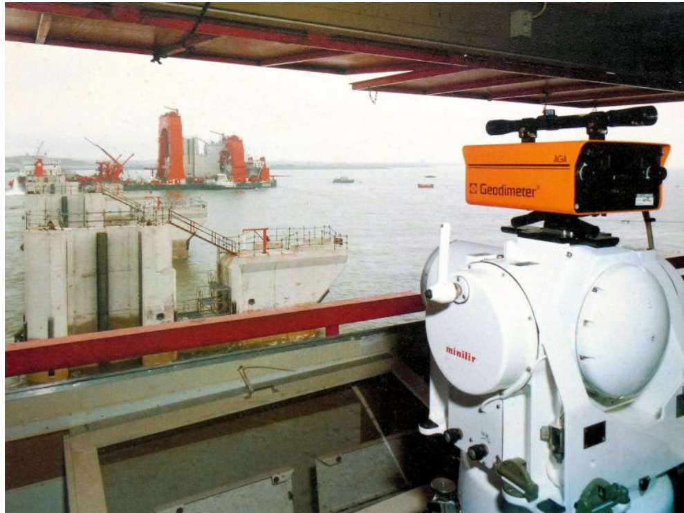
FIGURE 9.8. The AGA/Minilir infrared tracking device — French military technology! — in use on the building site of the Dutch Easter Scheldt storm-surge barrier, 1980. © 2016 Nicolàs de Hilster, (De Hilster), figure 4, with permission.
